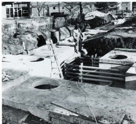
Concrete conduits are laid in trenches in front of Wismer Hall.
